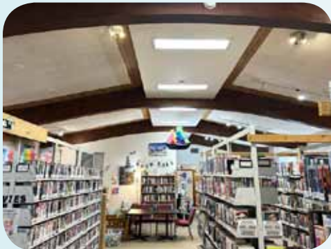
Interior - features glulam beams
