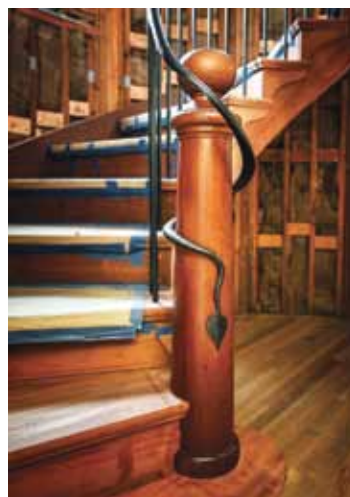
Smith Lake studio project newel post, with wrought-iron railing, designed by Ed and fabricated by regional blacksmith, Berkely Tack.
