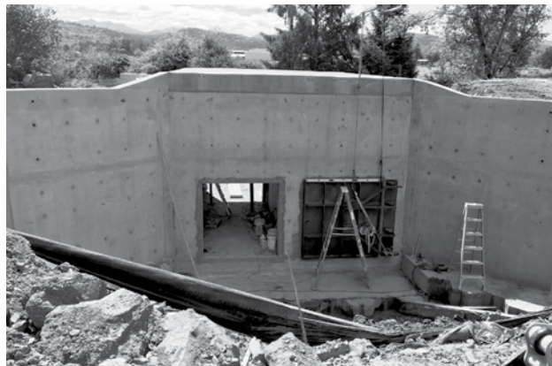
New tide gates nearing completion
